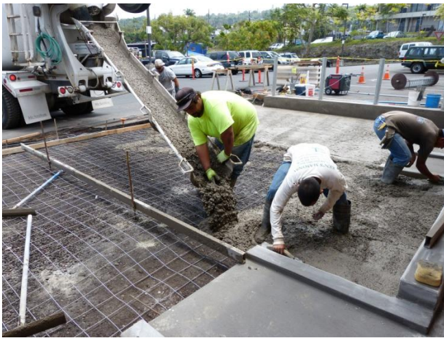
Placing of concrete
