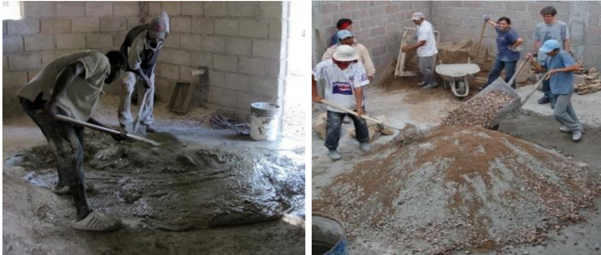
Manual mixing of concrete
