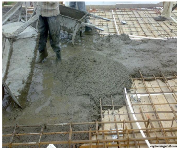
Placing of concrete
