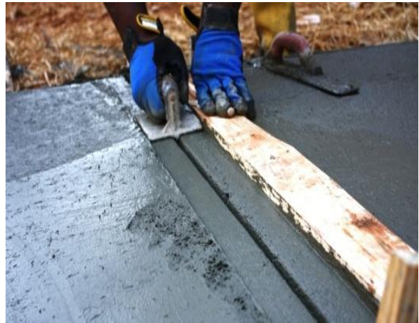
Groover (Grooving for joints)
